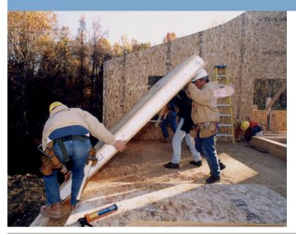
The basic design concept for SIPs is elegant in its simplicity, and offers several advantages for constructing walls and roofs. There is general agreement that SIPs provide better overall air tightness and practical thermal performance than conventionally framed walls.
